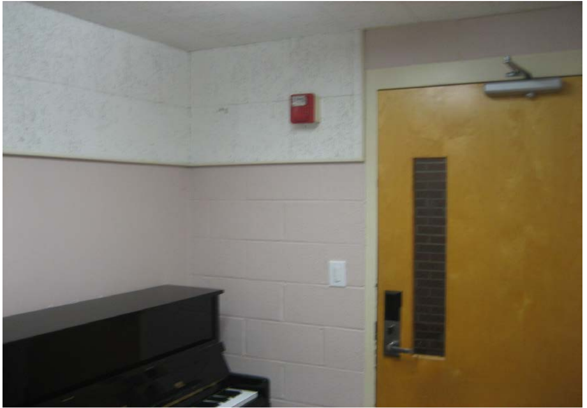
Practice rooms of original 1965 design have masonry corridor walls & acoustic panels adhered to a suspended ceiling. Typical gyp. board wall assembly between rooms has a n STC rating of 56.
