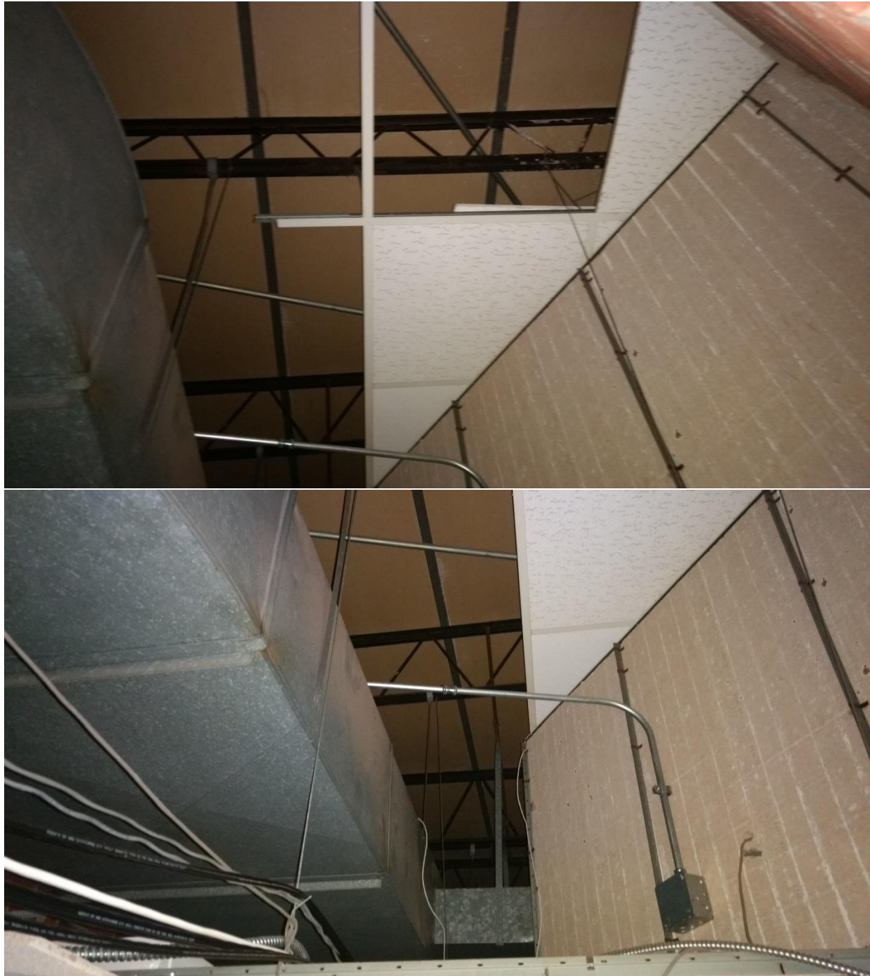
Figure 3: Area above ceiling outside choir room door (lifted acoustical ceiling tile just outside door)
