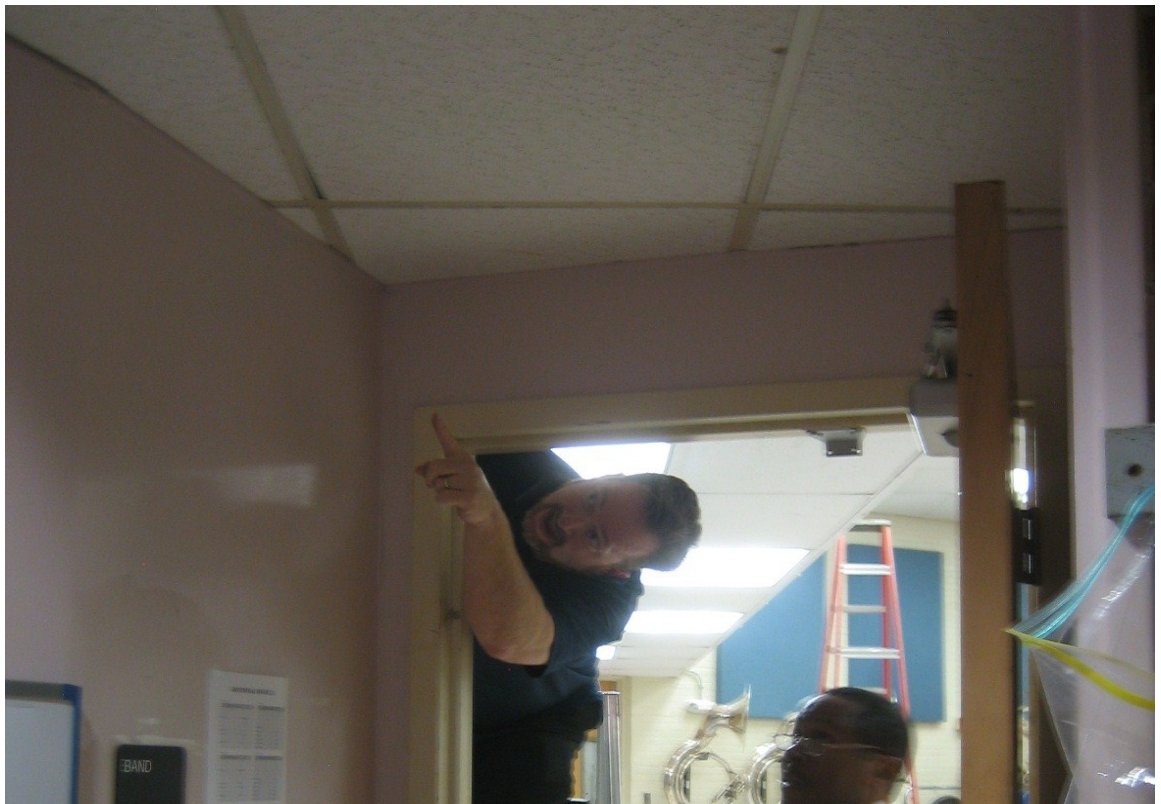
The recessed band room door is not original to the design and the walls above the suspended ceiling are incomplete creating poor sound isolation from the public corridor activities.
