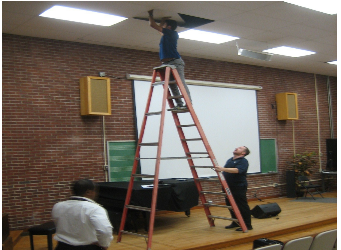
Inspection above ceilings is performed to confirm that room demising walls are sealed above ceilings to create proper room sound isolation.
