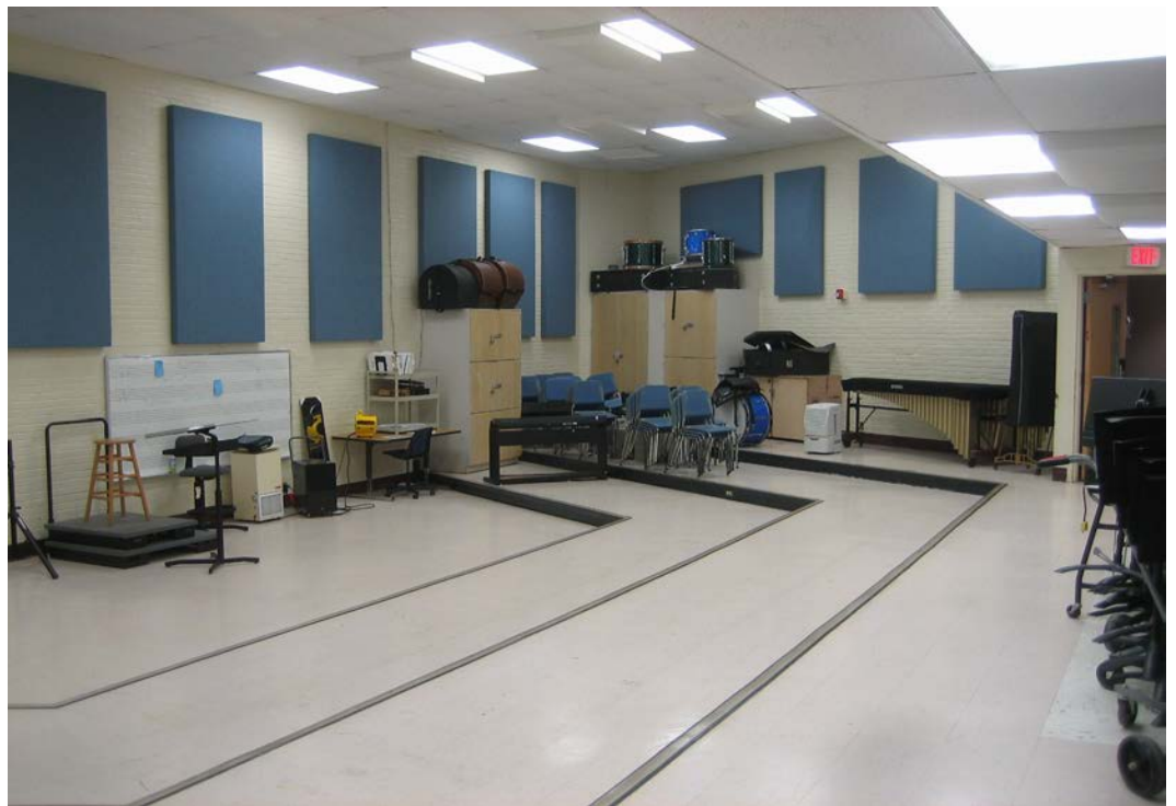
Band Room: Spatial volume, floor area, and ceiling heights are below minimum requirements based on the maximum occupancy of the room.
