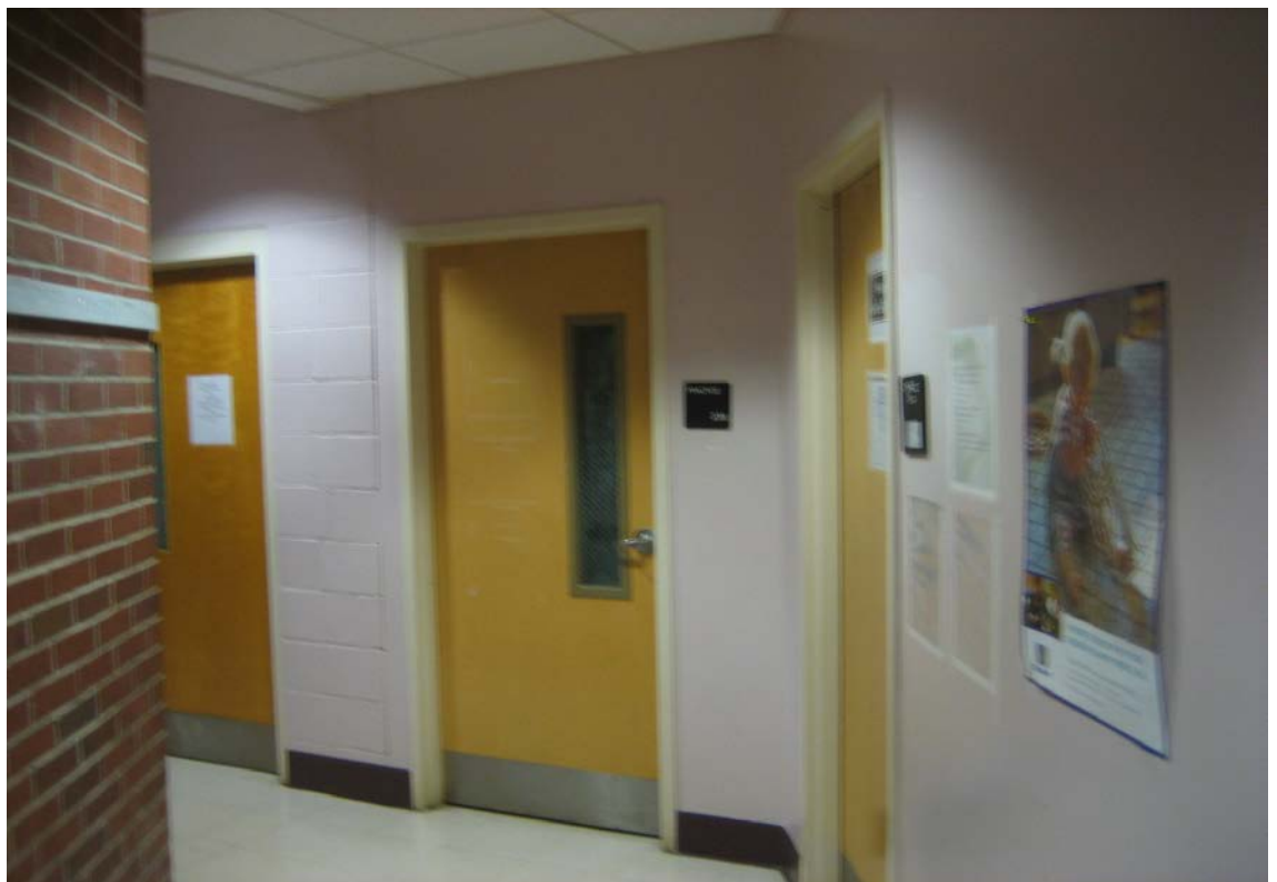
Corridor outside Chorus Room where original practice rooms concrete masonry walls join rooms renovated with gyp. board partitions creating ineffective sound isolation conditions.
