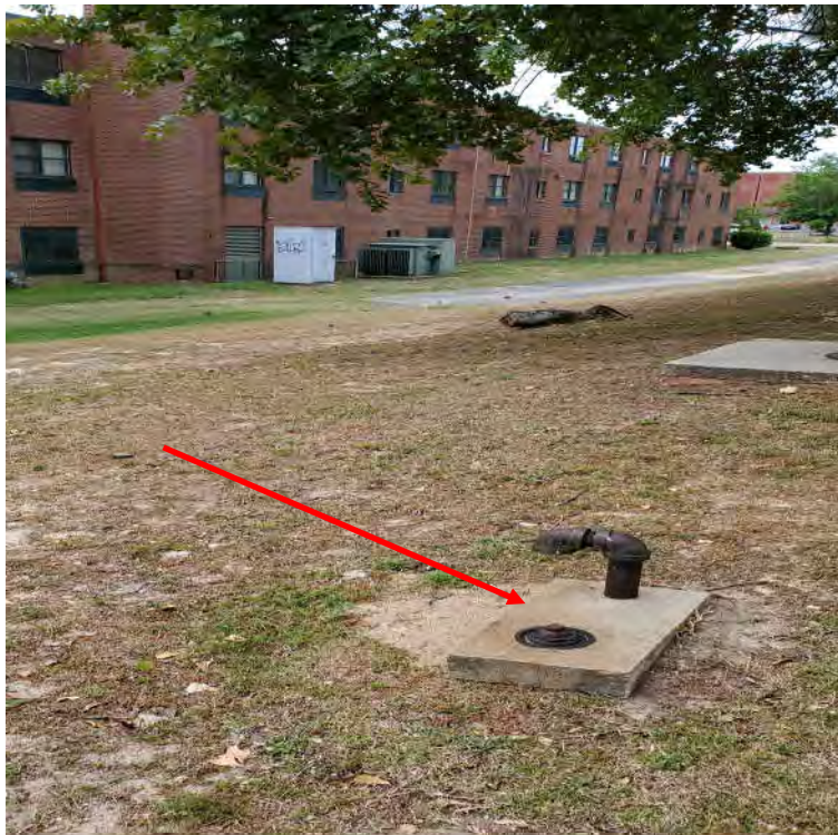
Photograph 8 - Suspect Underground Fuel Storage Tank (UST) Located at the Rear of Vance Hall.
